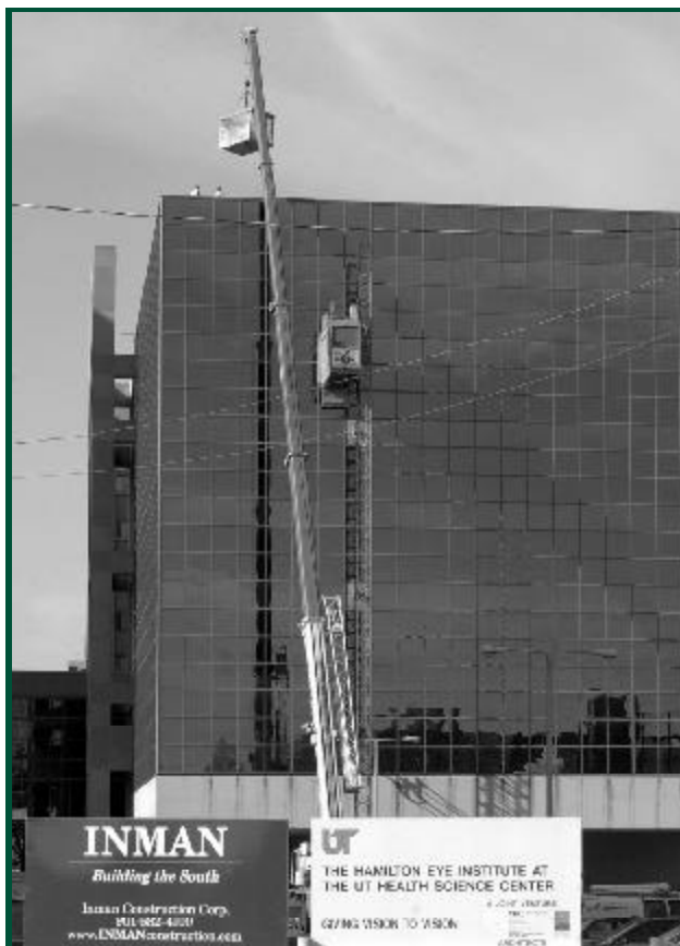
THE HAMILTON EYE INSTITUTE UNDER CONSTRUCTION
